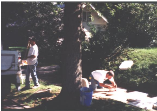
Repair in progress, Jackson St.
