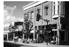
Downtown Flagstaff after streetscape improvements.
